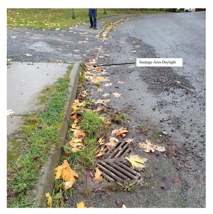
Photo H: Storm drain catch basin fed by seep at edge of gravel driveway. Facing southeast.
