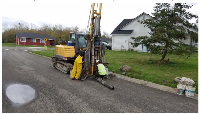
**Photo B:** Site of borehole B-2 on the north side of Alphonsus Bob Loop Road. Pavement cracking and utility trench subsidence with water in pothole at lower left. View facing west.
