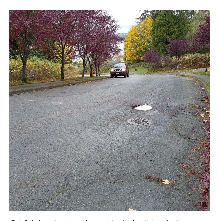
**Photo B:** South-central roadway area showing pothole and cracking. Facing northwest.
